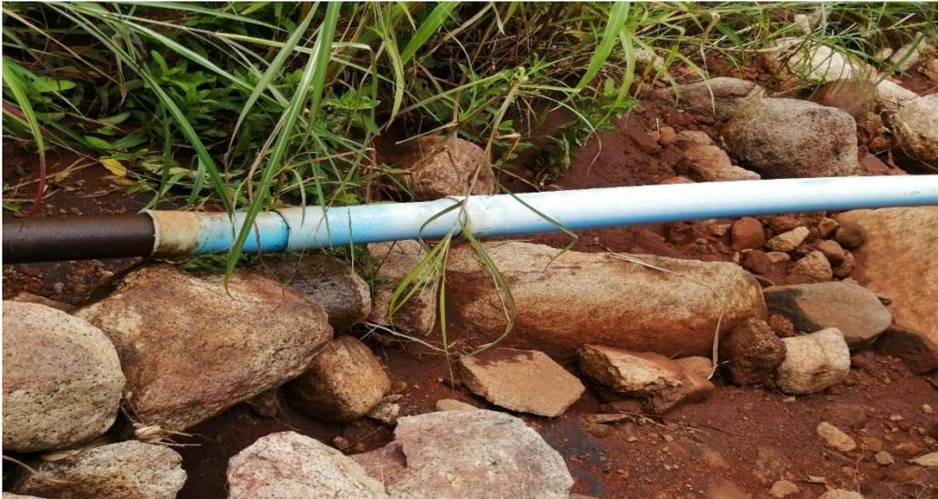
**Figure 3: Maintenance using old materials.**
