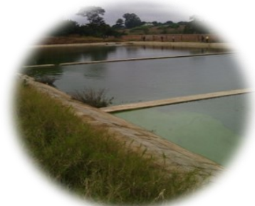
MZUNI Wastewater Treatment Plant (WWTP)
